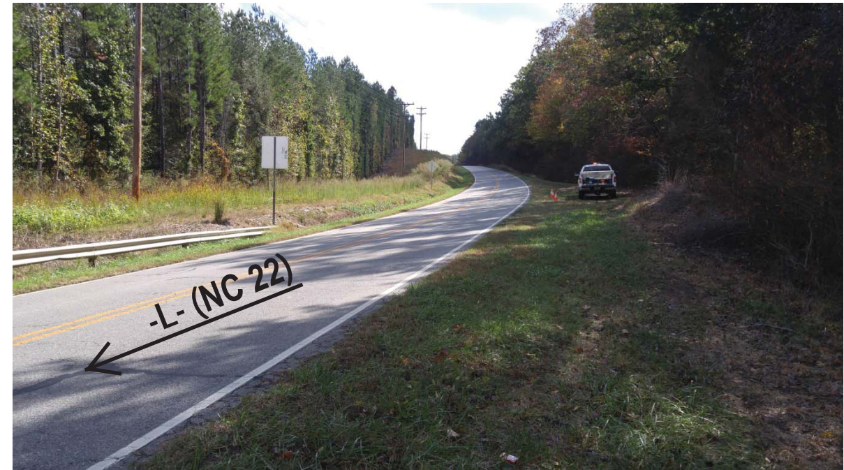
Looking Southeast along NC 22
